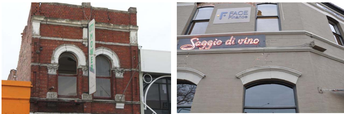
(a) Extensive vertical cracking above window openings
