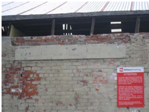
(b) Side-view of tilted joists
