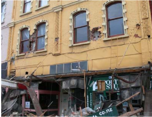
(a) Anchorage failure
