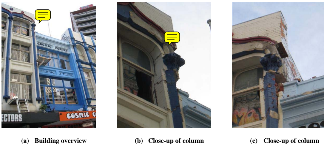
Figure 3.22 Example of building pounding damage
