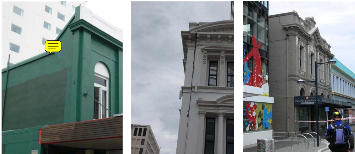
Figure 3.21 Examples of wall separation at corners of buildings
