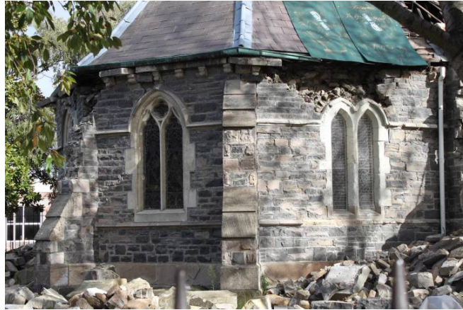
Figure 3.43 St. John's the Baptist Church. Local collapse of material
