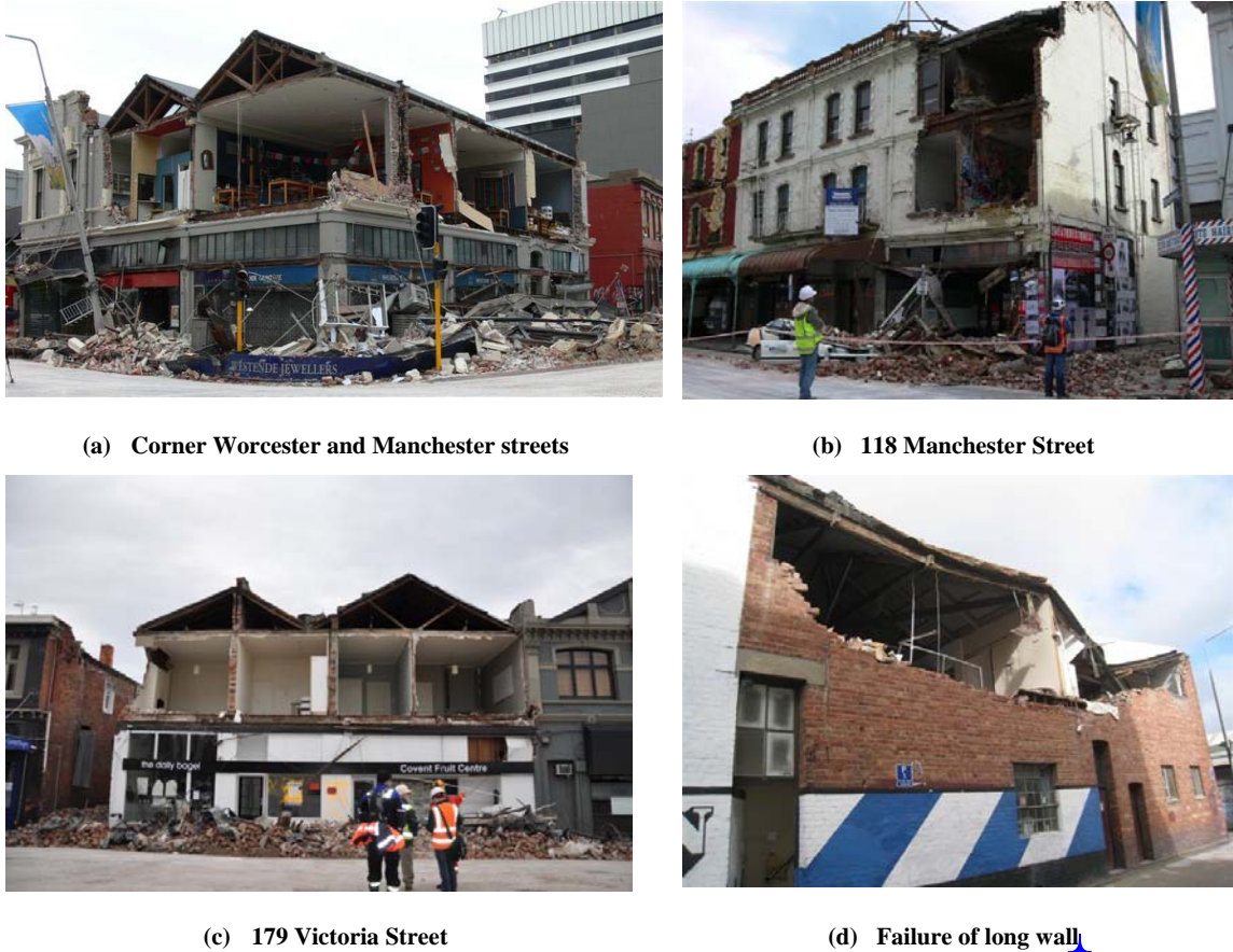
Figure 3.10 Examples of out-of-plane failures in solid masonry walls
