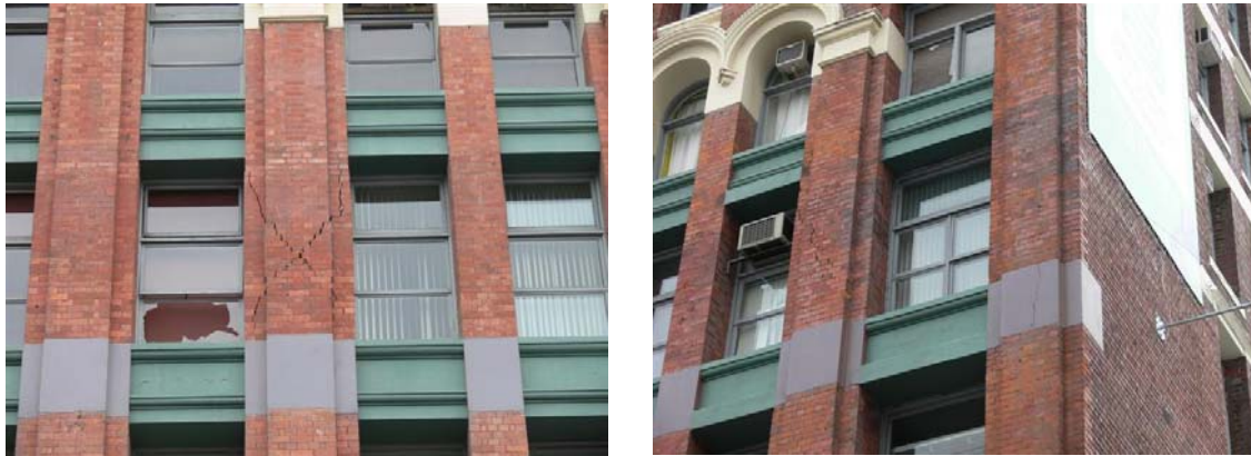
(a) North wall piers, levels 3-4
