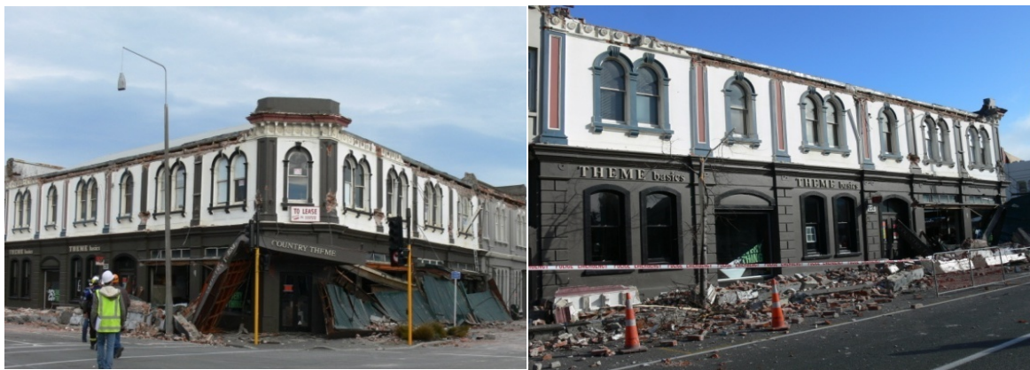
(a) Corner view showing parapet collapse
