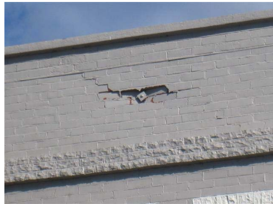
(b) Detail of partial anchorage failure
