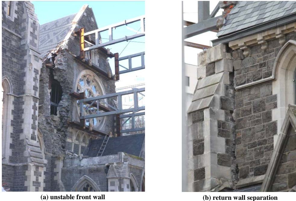
Figure 3.30 Christchurch Anglican Cathedral – front façade damage
