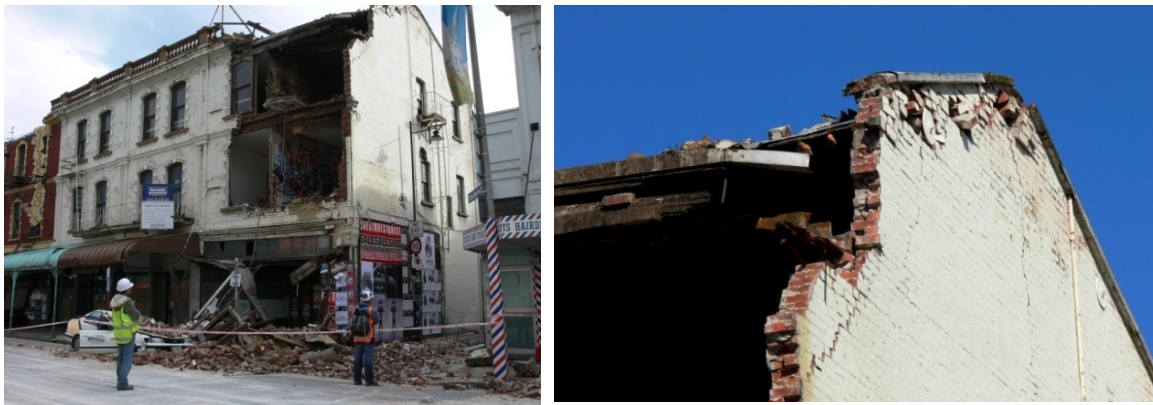
(a) 135-139 Manchester Street, out-of-plane facade collapse
