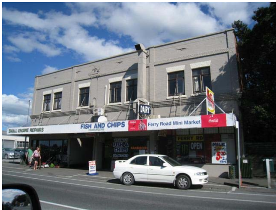
(a) Building overview
