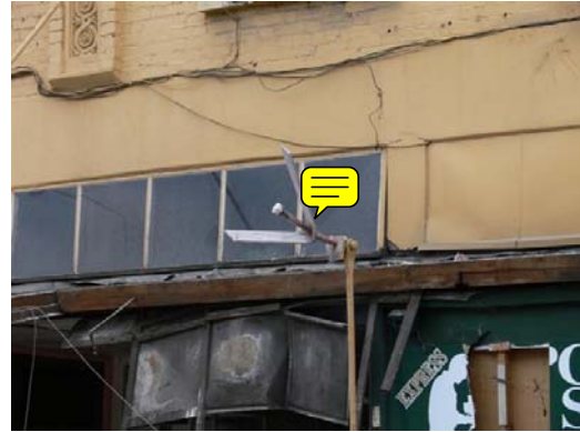
(b) Close-up of failed anchorage detail
