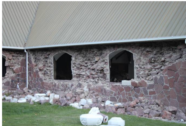
Figure 3.42 Lyttelton Holy Trinity Church. Damage induced by hammering of the roof
