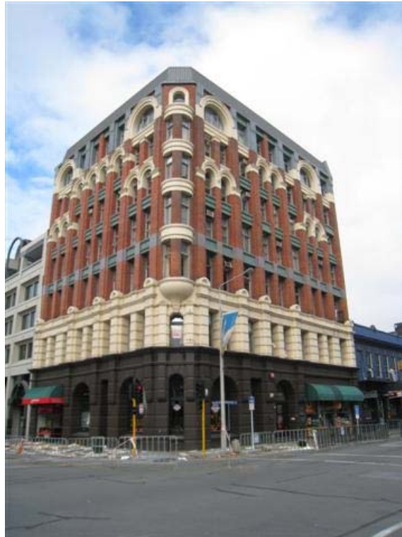
Figure 3.23 Manchester Courts building (view from NW)
