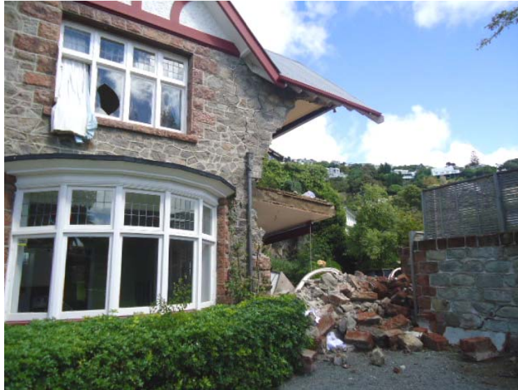
Figure 3.31 Rockvilla dwelling with complete collapse of the north and east façades
