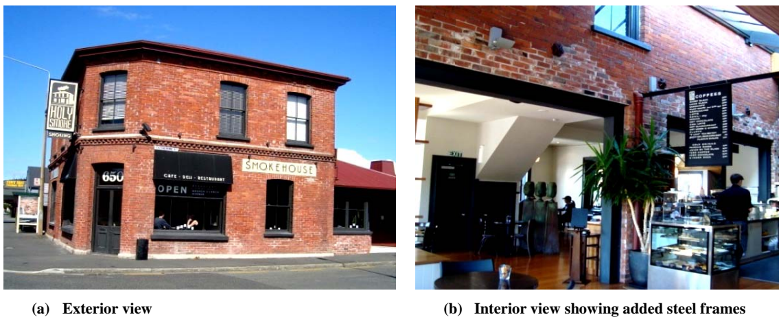
Figure 5.6 The Smokehouse, 650 Ferry Road (images taken post-September 2010)
