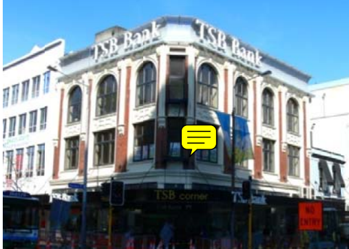
(a) Exterior view
