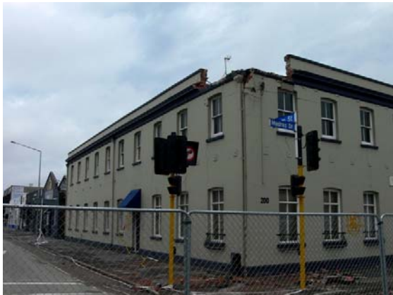
(b) Exterior view of failed parapet at corner
