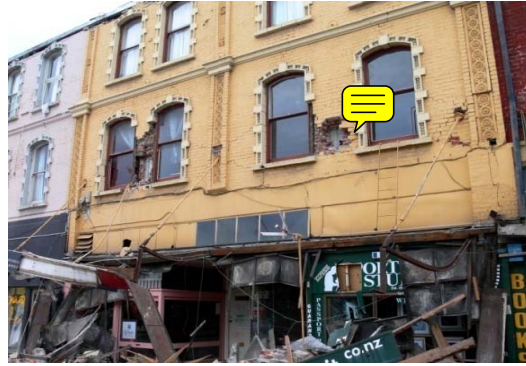
Figure 5.15 137 Manchester Street, pull out of the canopy supports
