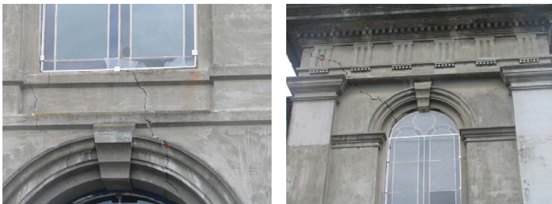
(c) Vertical crack through spandrel
