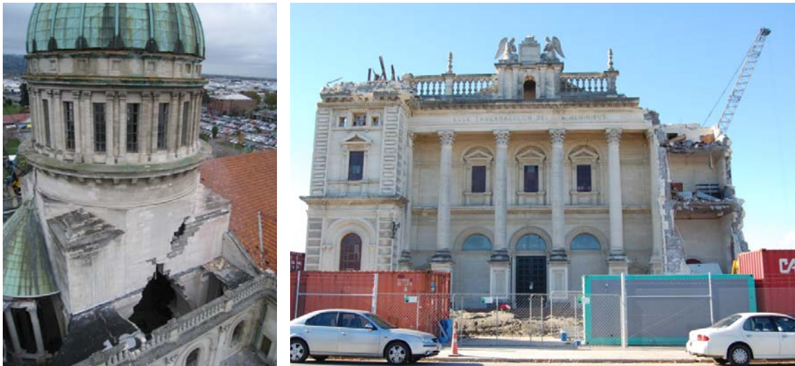
(a) Damage to drum at base of dome
