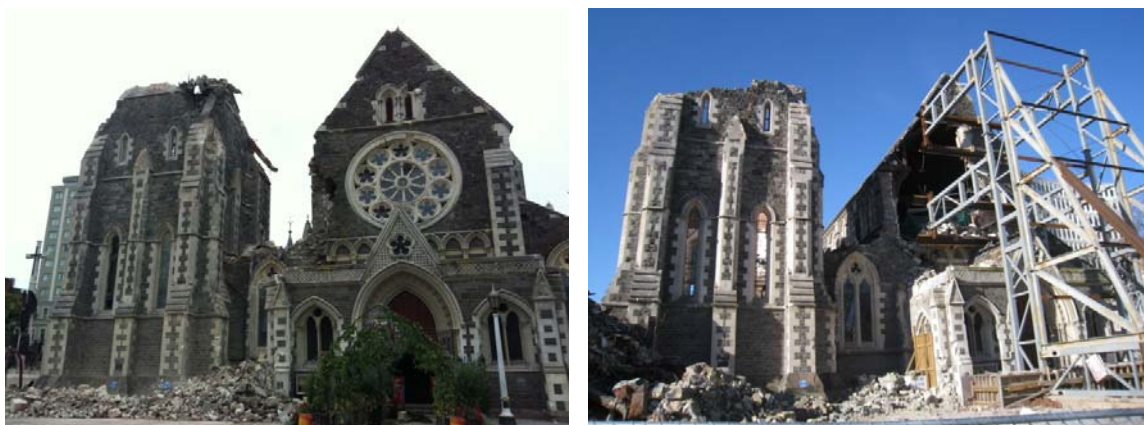
(a) Condition after 22 February 2011
