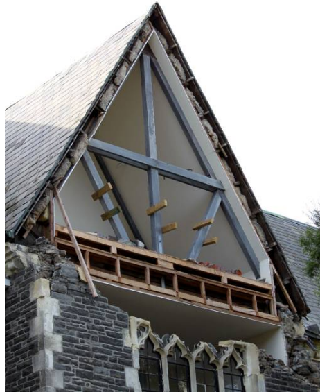
Figure 3.33 Cramner Court, showing complete collapse of a gable
