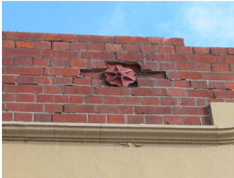
(a) wall-diaphragm anchor punching
