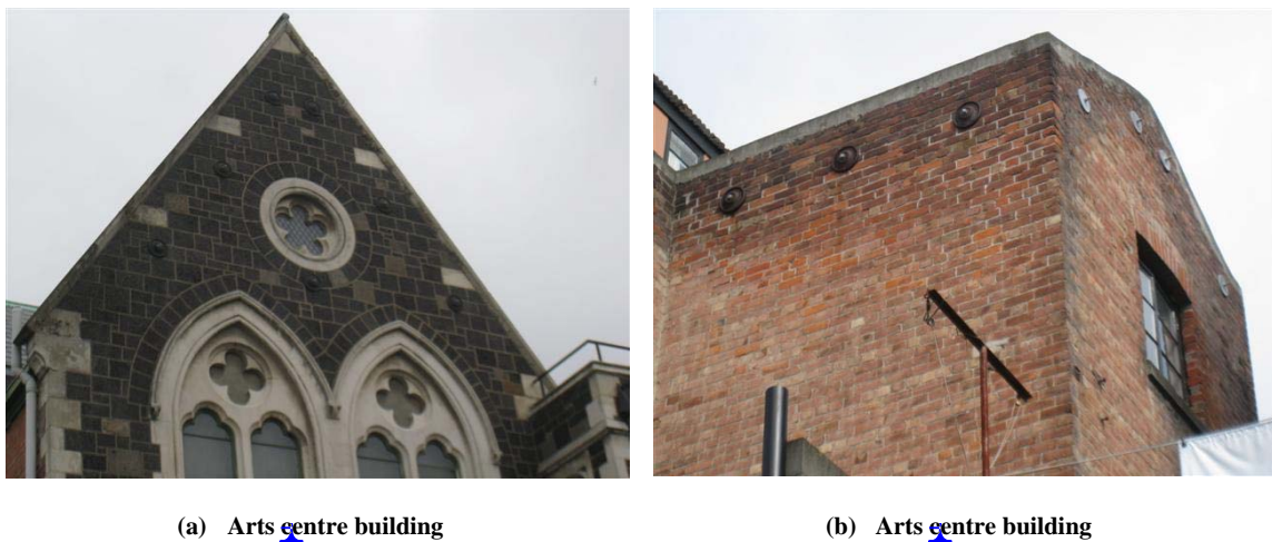
Figure 3.14 Successful gable end wall and side wall anchorages
