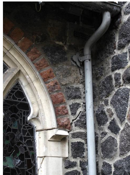
(b) Exterior view
