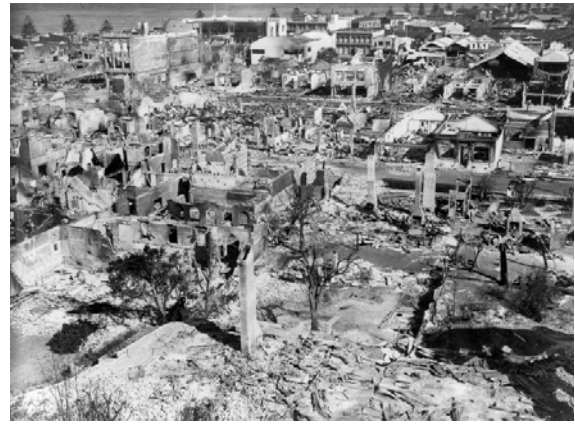
(b) Overlooking Napier at the buildings ruined by the 1931 earthquake and the fires [Alexander Turnbull Library]
