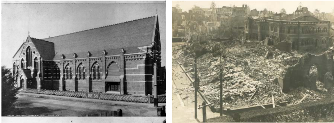
(a) St John's Anglican Cathedral in Napier, ca. 1885 [Alexander Turnbull Library] (b) Ruins of the Napier Anglican Cathedral after the 1931 Hawke's Bay earthquake [Alexander Turnbull Library]
