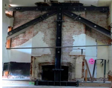
(b) steel brace frame
