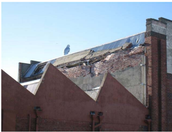
(c) Side wall parapet collapse onto roof.
