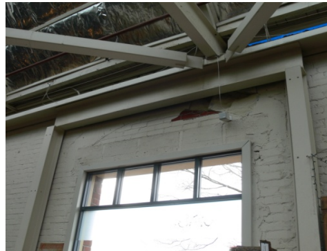
(c) interior of the building (location where anchor plate pull out occurred)
