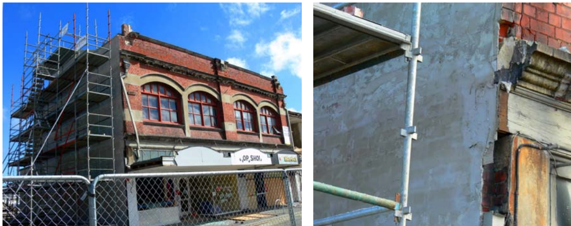
(a) Exterior view of retrofitted building
