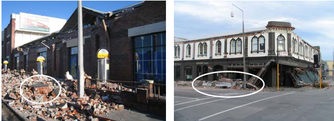
(a) Solid section of masonry gable
