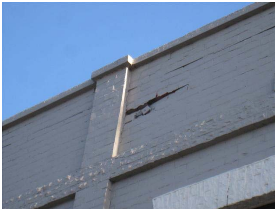
(c) Onset of anchorage failure
