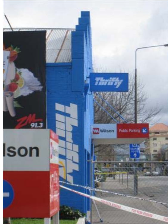
(c) Front wall curvature
