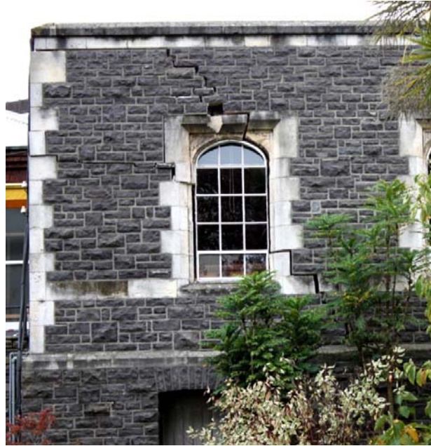
Figure 3.35 Canterbury Provincial Chambers - diagonal crack through entire south façade of the east annex
