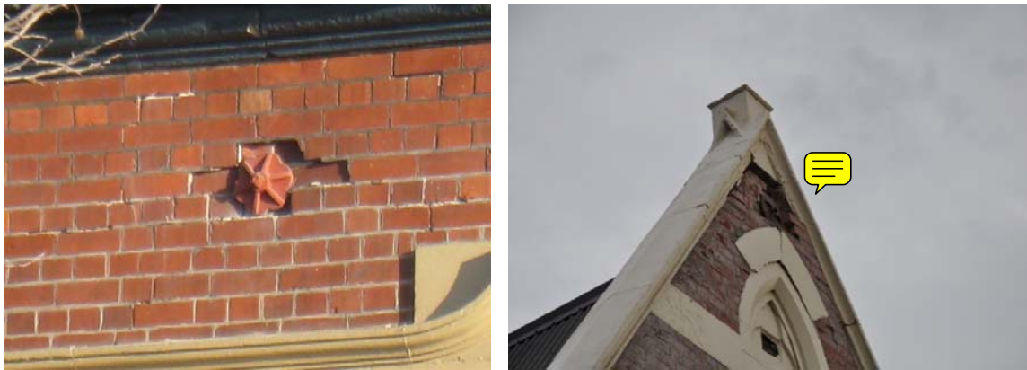
(a) Wall-roof anchorage failure
