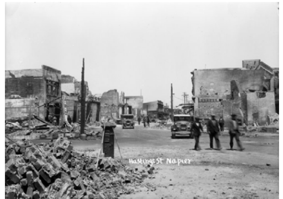
(d) View down Hastings Street, Napier after the earthquake 1931 [Alexander Turnbull Library]
