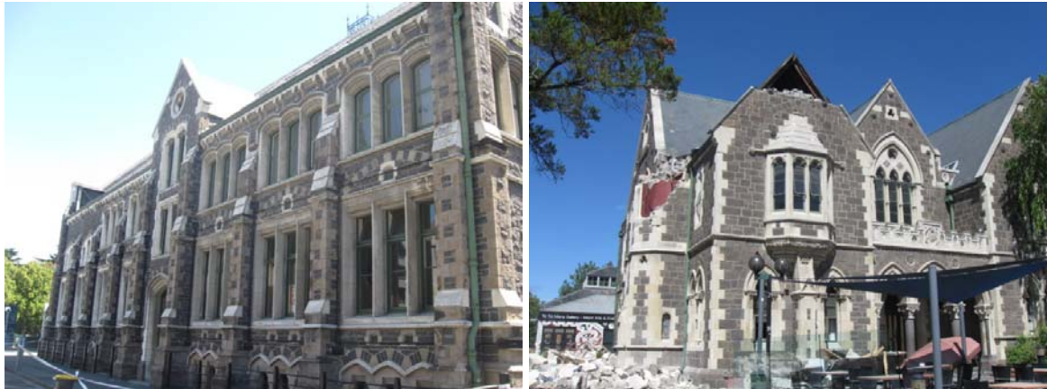
(a) Good performance of stone masonry building with horizontal and vertical external post-tensioning
