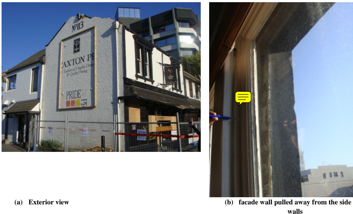
Figure 5.21 Caxton Press building at 113 Victoria Street (images taken post-September 2010)
