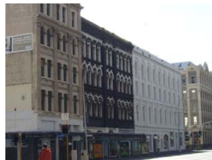
Typology F building – three+ storey row
