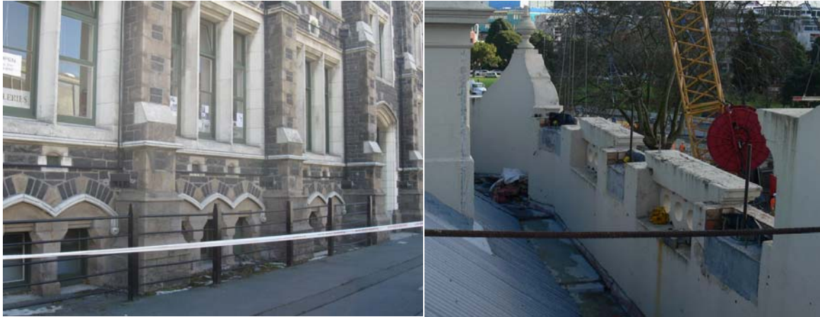
(a) External post-tensioning used in the Christchurch Arts Centre (photo taken after 22 February 2011 earthquake)
