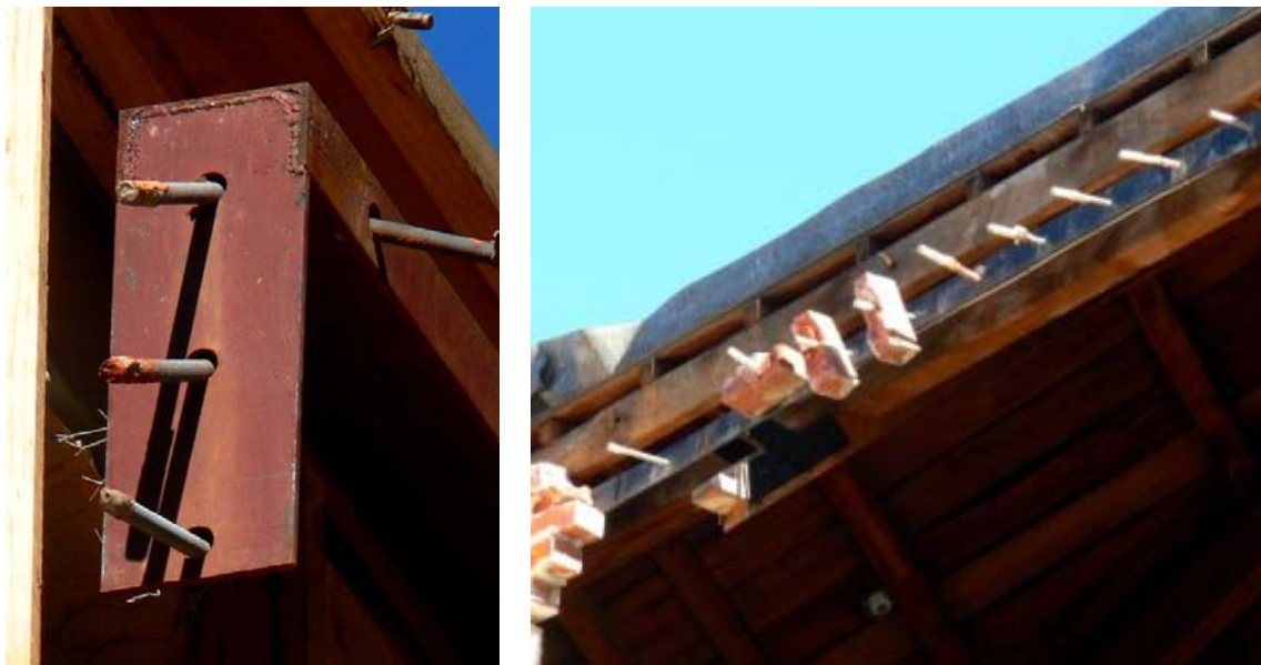
(a) Failure of a steel fixing due to anchor withdrawal
