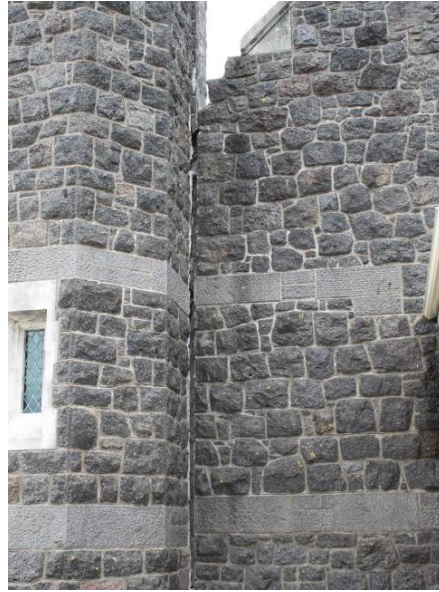
Figure 3.37 St. Mary's Anglican Church - detachment of the bell tower from the nave
