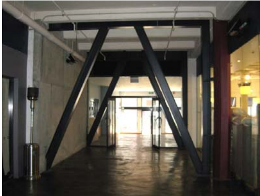
(a) Eccentric bracing in a walkway
