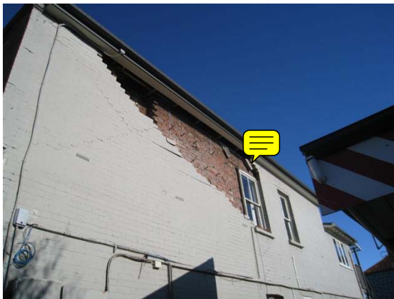
(c) Butterfly wall ties still intact
