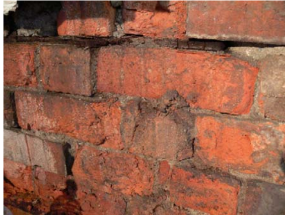
Figure 4.2 Severely degraded bricks and mortar due to moisture ingress
