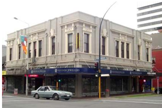
Figure 5.19 Welstead House, 184-188 Manchester Street, before the 4 September 2010 earthquake
