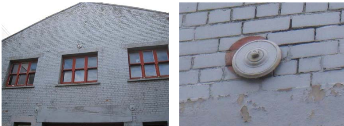
(a) Overview of wall anchors
