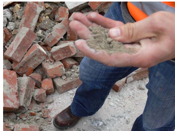
(b) Weak mortar crumbles between fingers
