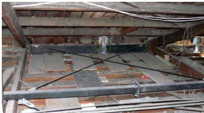
(e) roof diaphragm strengthening
