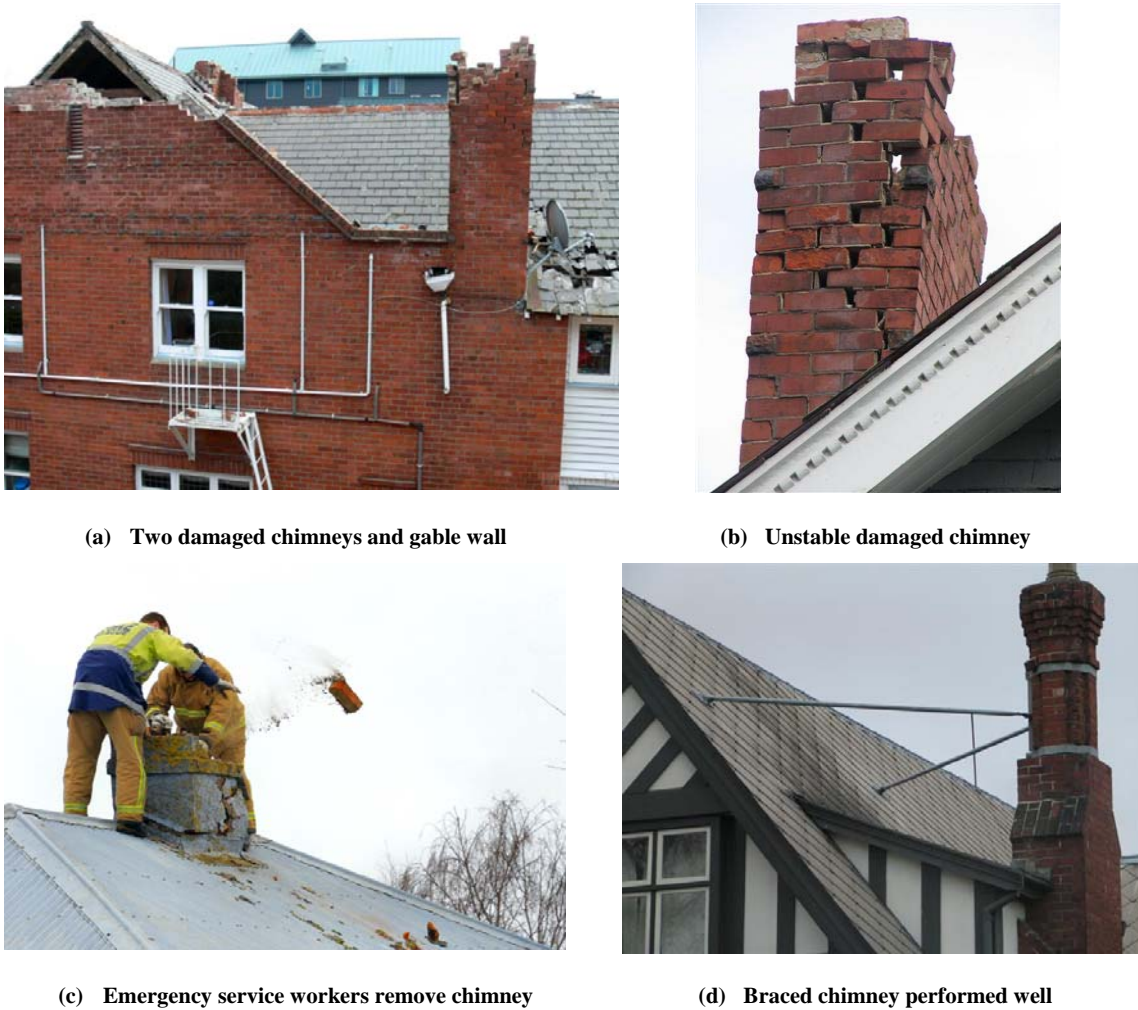
Figure 3.6 Examples of chimney performance during the Darfield earthquake
