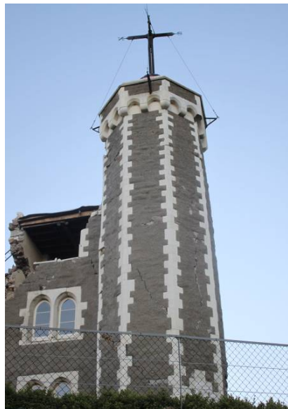
Figure 3.44 Time Ball Station. Damage in the Time Ball tower
