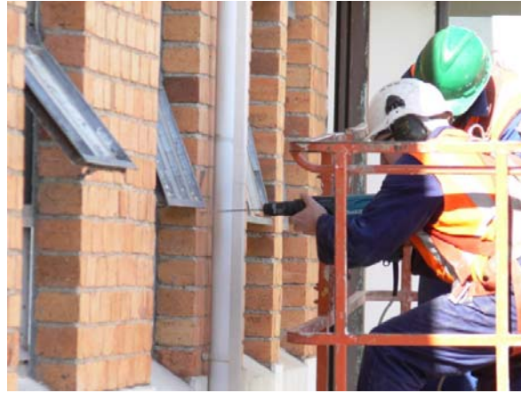
Figure 4.6 Use of drilled ties to fix external leaf to internal leaf
