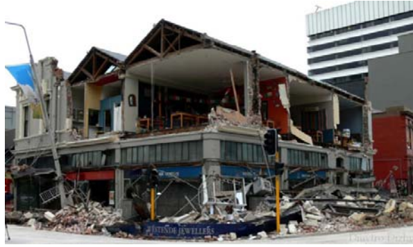
Figure 4.10 An extreme case in the 2010 Darfield earthquake where inadequate connections have resulted in wall collapse (Welstead House, 184-188 Manchester Street)
