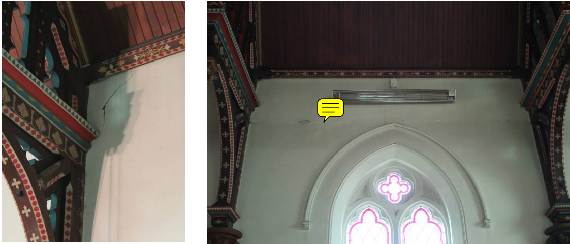
Figure 3.41 St James' Church, hammering of roofing elements on the walls of the nave
