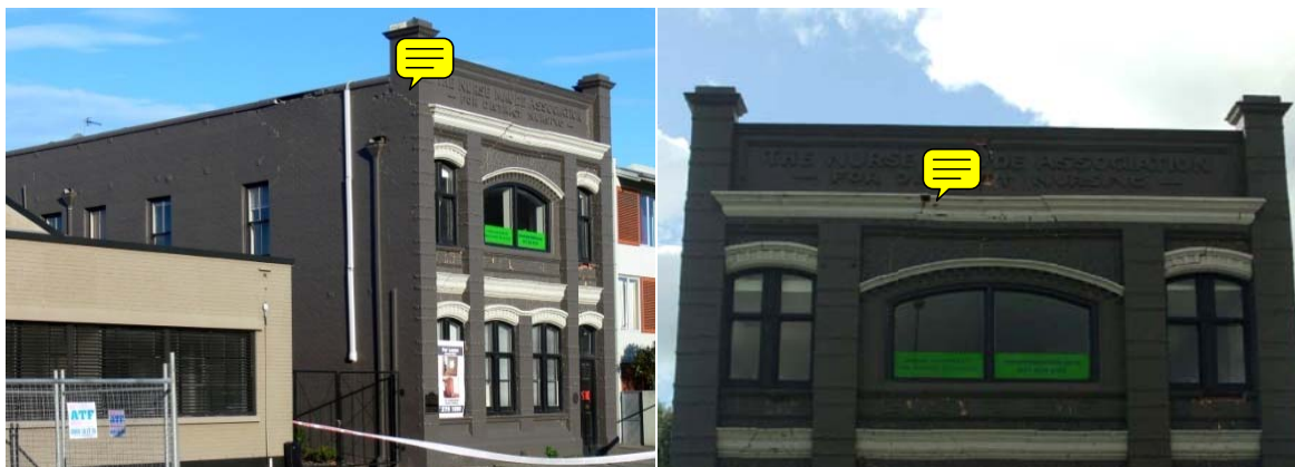
(a) cracking through top spandrel
