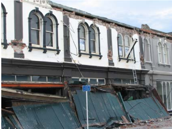
(a) Multiple front wall parapet failures
