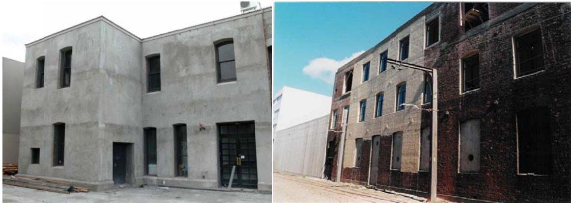
(a) Shotcrete applied to a former URM building
