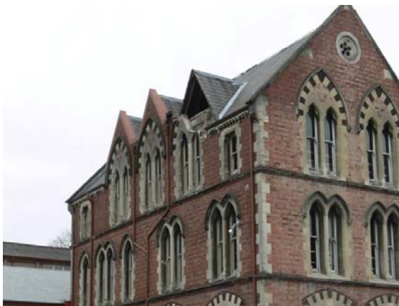
(c) Montreal-Armagh street corner
