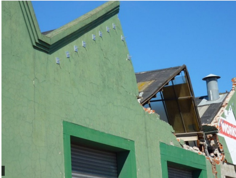
Figure 4.1 Example of a secured gable end that survived earthquake loading and a companion failed gable end that was not secured
