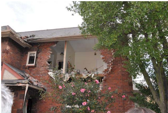
(a) Cavity wall failure in a residential building
